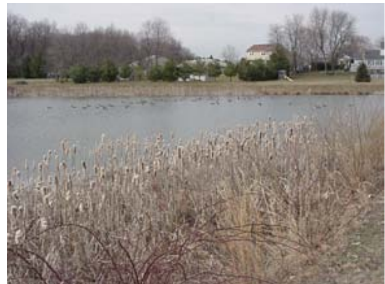
Pigeon Run Stormwater management basin beautifies the County's drainage effort.
